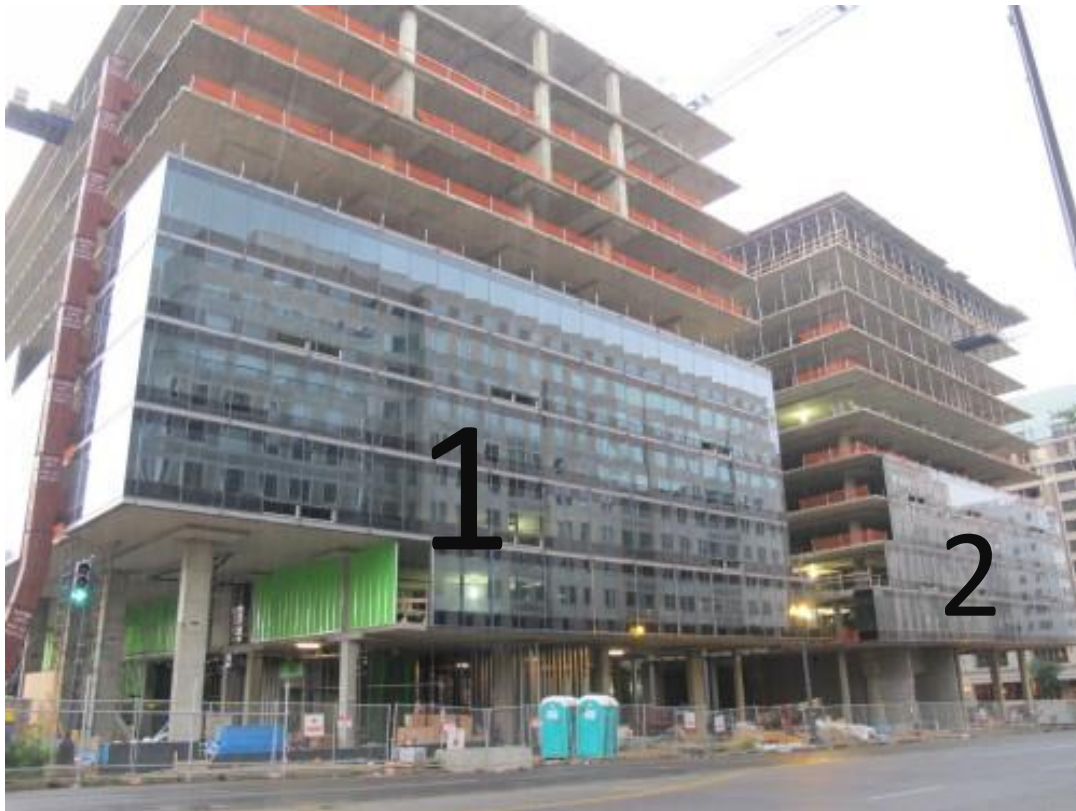
Figure 3.1: Construction of One and Two City Center with structure exposed.
