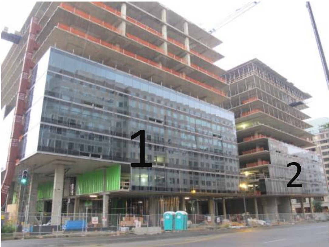
Figure 3: Construction of One and Two City Center with structure exposed.
